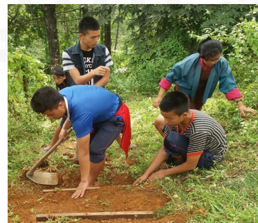
YCS students construct footpath to boys hostel.
